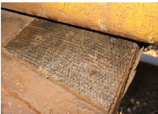
Carrier Plate Fibrous Material Containing Asbestos Wear Liner
