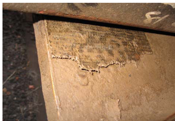
Fibrous Wear Liner in Poor Condition To be Removed from Service
